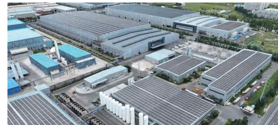
PV Wafer Manufacturing Base
