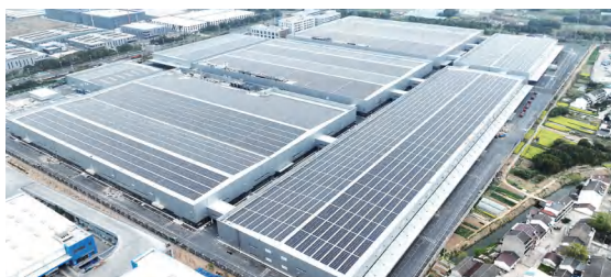
PV Module Manufacturing Base
